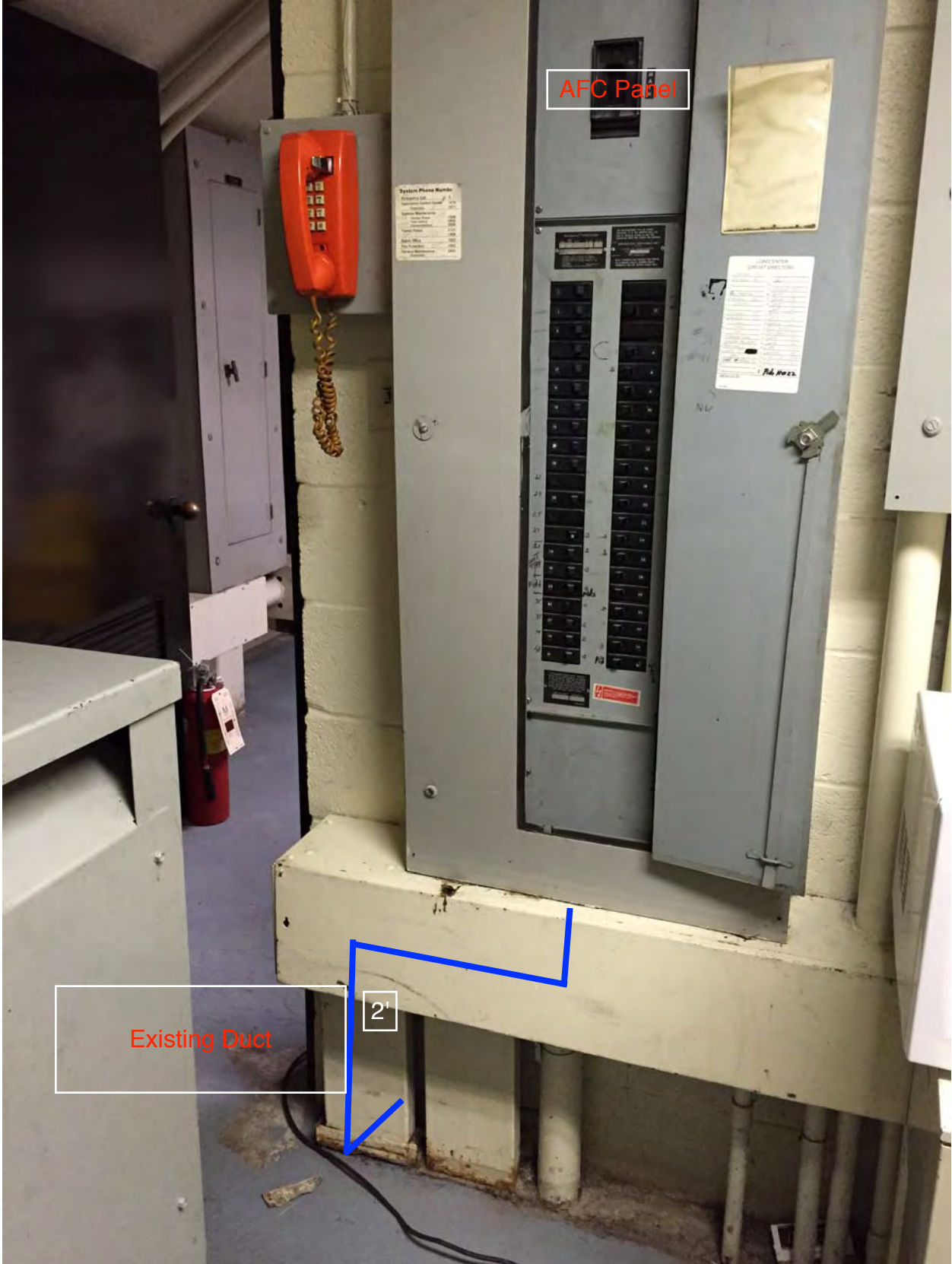
Photo #4: Existing duct route
